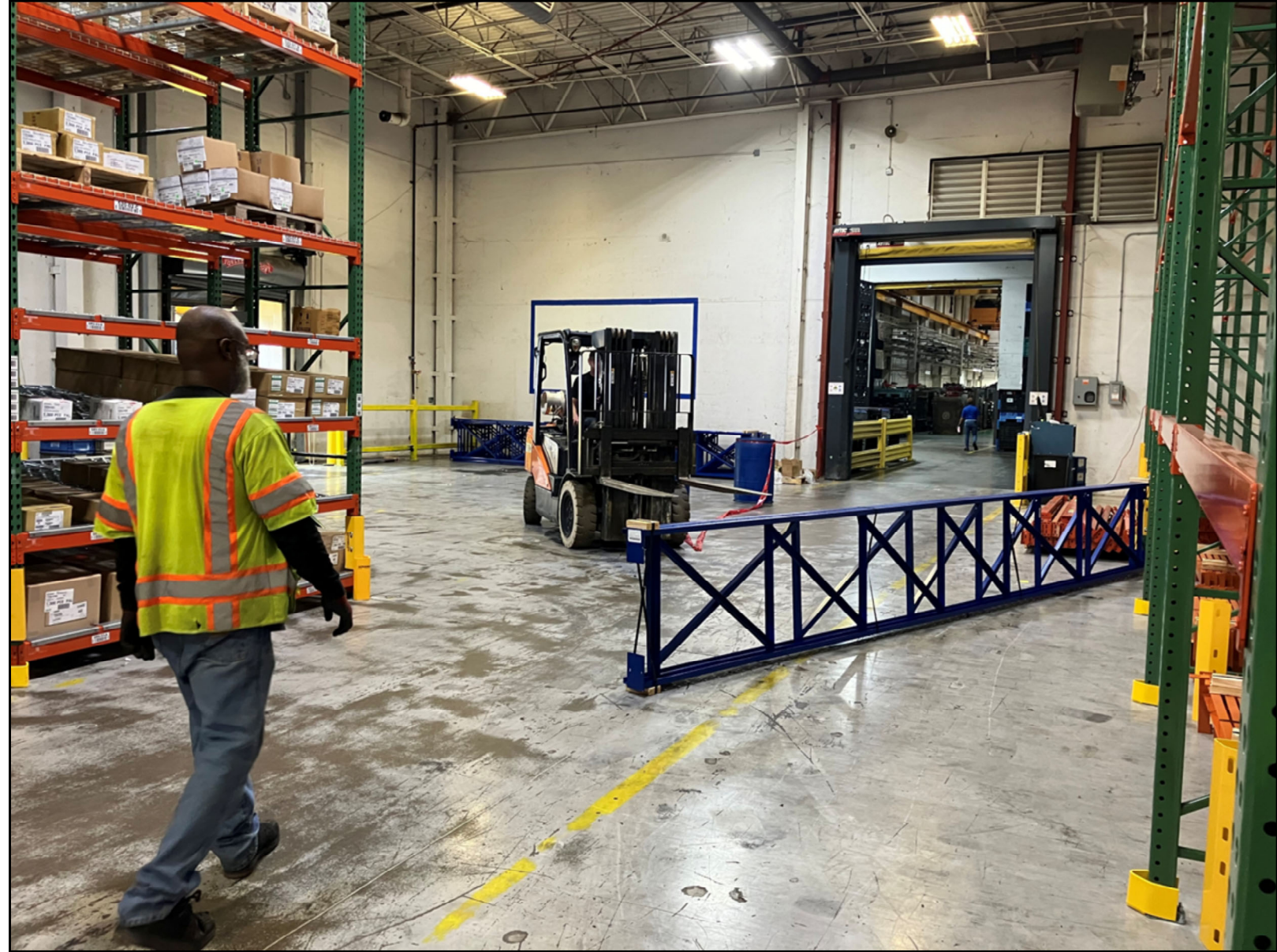
Progressive installation slide 12. Installation of drive-in racking system.
