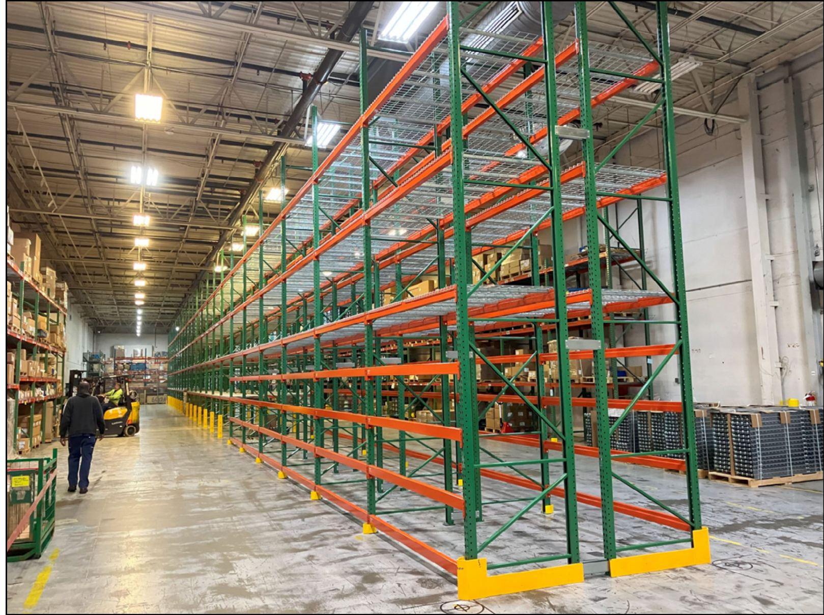
Progressive installation slide 11. Foreground is the gravity flow rack.
