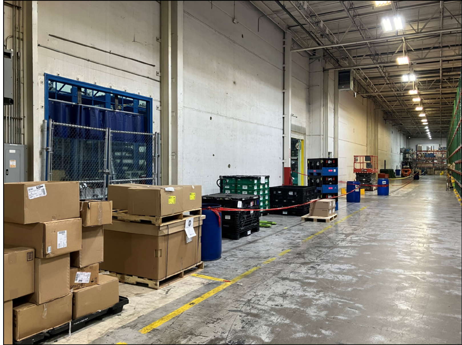
Preparation for the installation.
