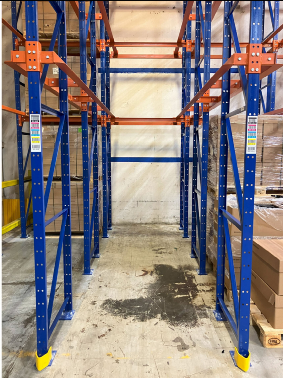
Progressive installation slide 14. Finished installation of the drive-in racking system. Bar coded signs installed.
