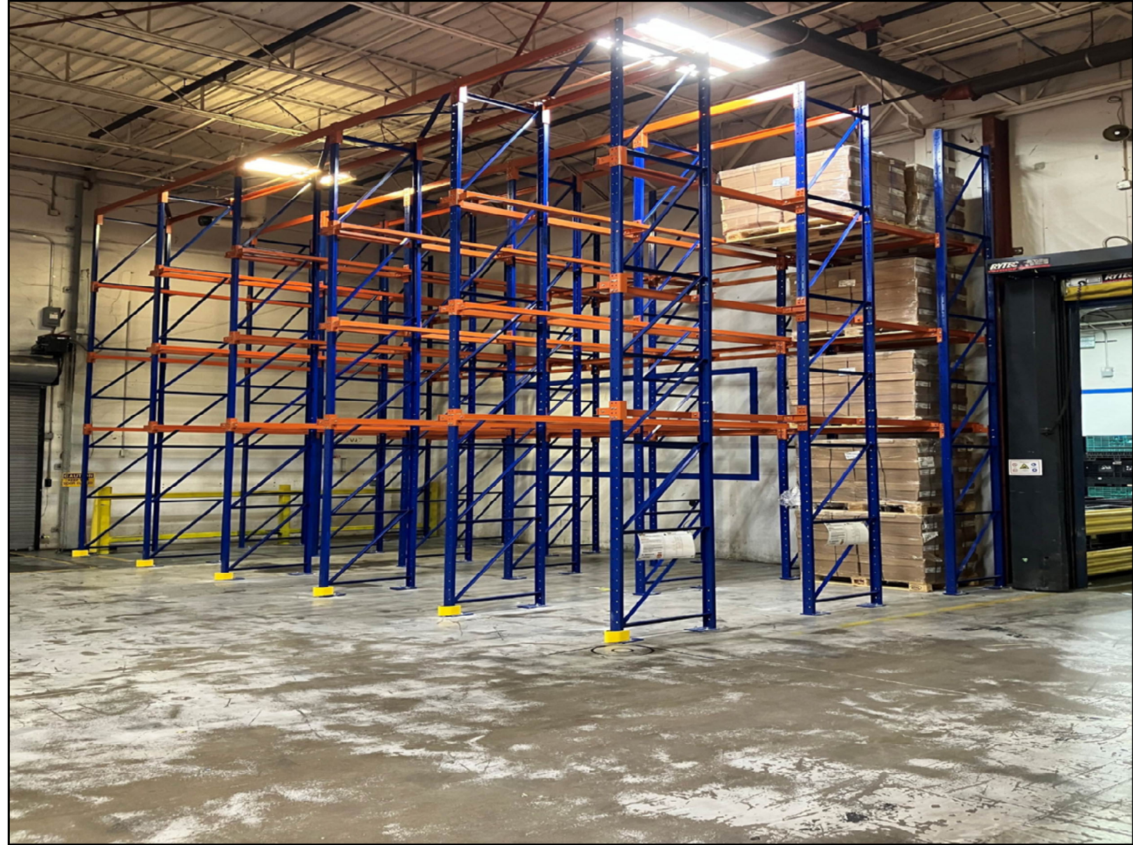
Progressive installation slide 13. Installation of drive-in racking system completed.
