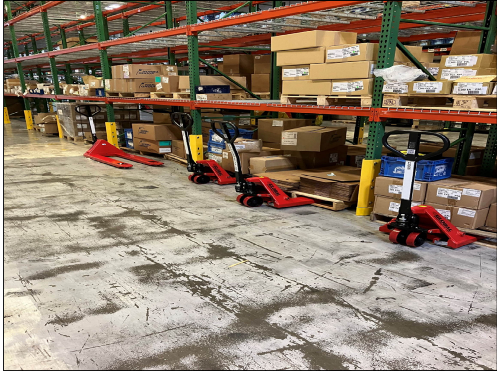
Progressive installation slide 17. Installation of drive-in racking system.
