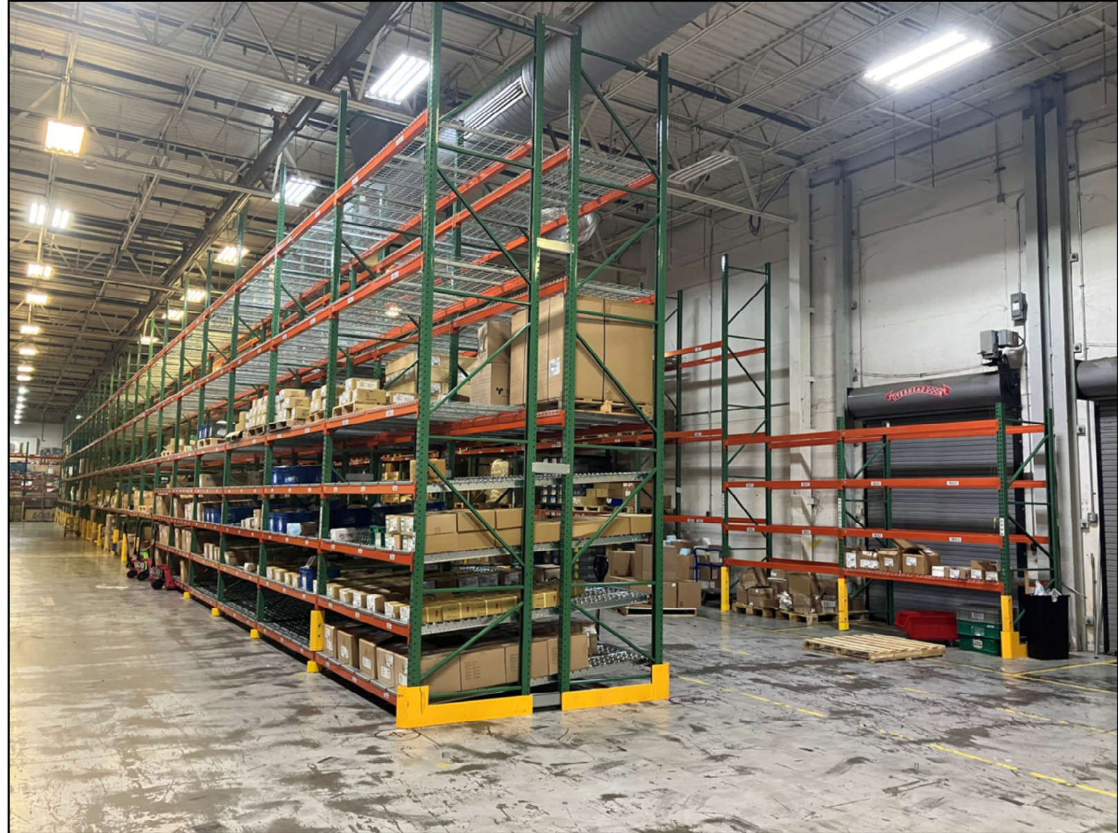
Progressive installation slide 8. Flow rack installation completion.
