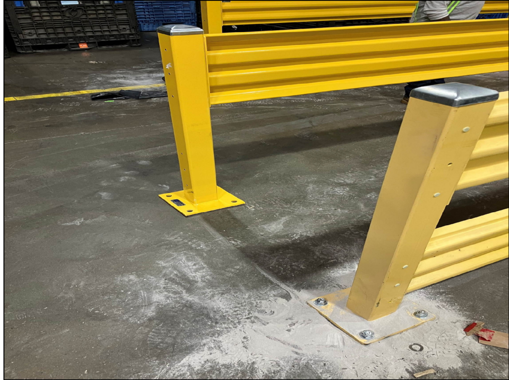
Progressive installation slide 15. Pedestrian guard rails installation.
