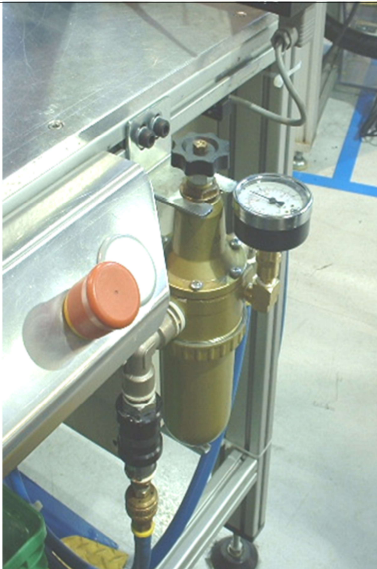
Making gauges easier to read by my installing a 90° degrees elbow...
